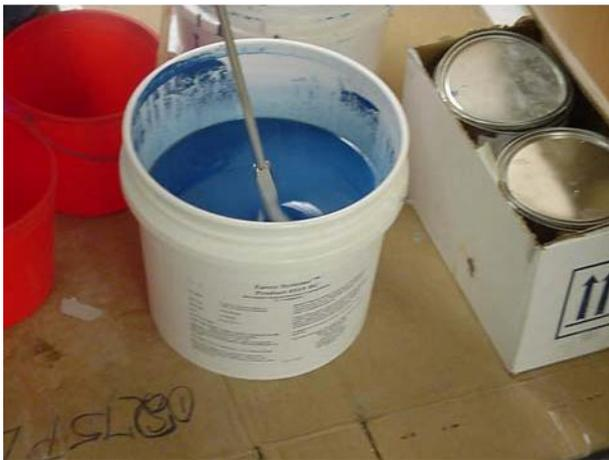
Stir the Resin “A” and the Hardener “B” each separately in their original container before measuring and mixing the two together. Be careful to use separate stir sticks so not to cross contaminate.
